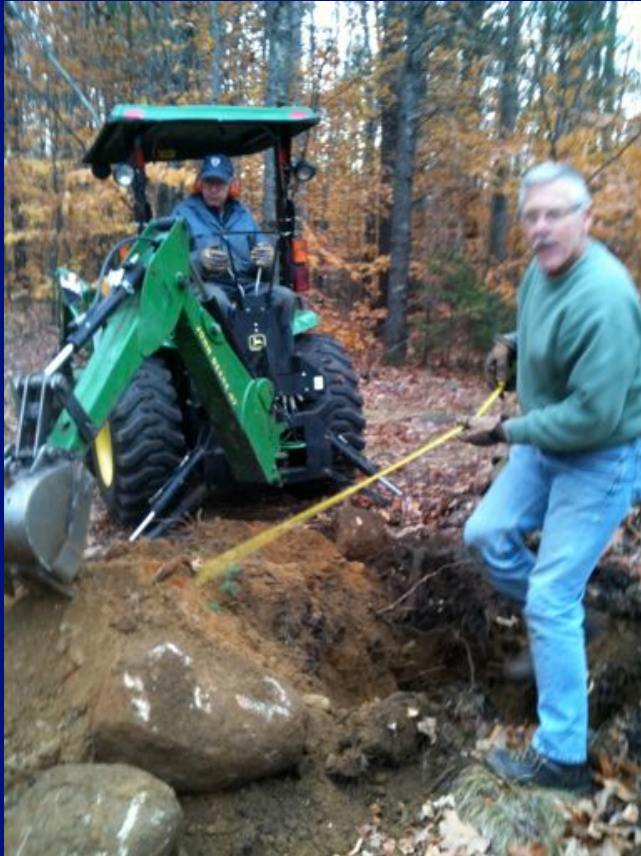
Erosion control work, Page Hill Trail, October 2010
