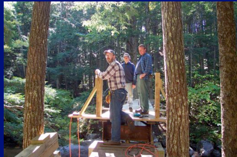
Rebuilding the bridge over Swift River at Big Pines Natural Area, 2002
